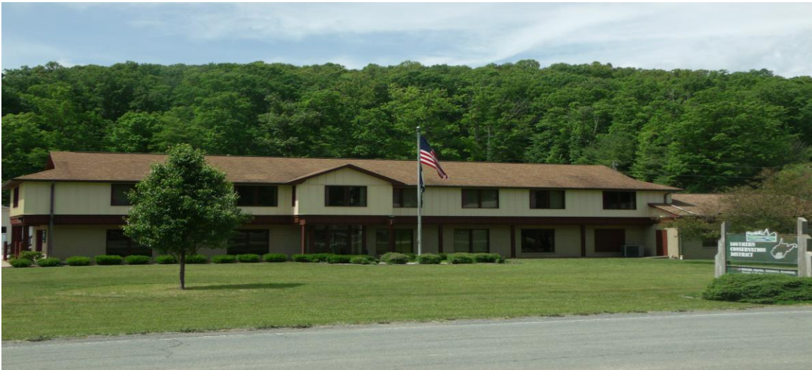
SCD Building, 463 Ragland Road, Beckley, WV
