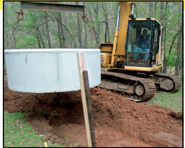
The TVCD crew sets a 400 gallon watering trough. Our district sells these and other troughs and float parts.
