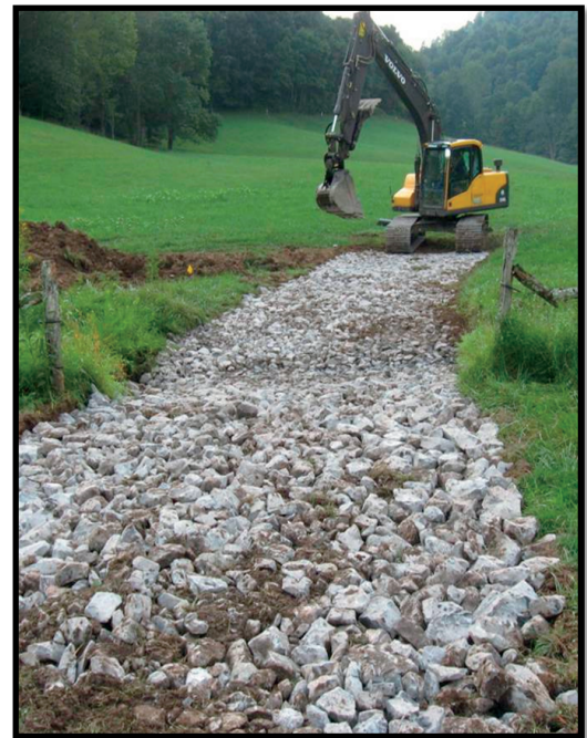
Installation of a Heavy Use Protection Area. By laying rock and gravel down atop filter fabric, this heavy use area will no longer be flooded after heavy rain and will allow for better traction for vehicle use.
